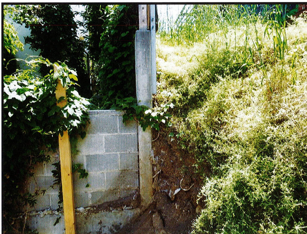
Photograph 8 – Photograph captured 19 November 2020. View of the western end of the subject land, looking west, at the north-east corner of 1 Campbell Grove (north-east corner of 1A Campbell Grove). Note vertical face of earth adjacent to concrete retaining wall.
