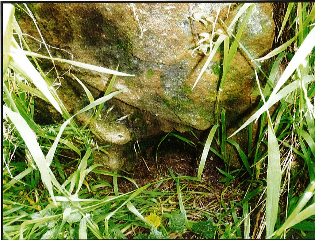
Photograph 16 – Photograph captured 13 October 2021. View of rock outcrop along the southern side of the subject land (i.e. long 1 Campbell Grove boundary). No evidence of loose / displaced soil at the toe of the rock outcrop.
