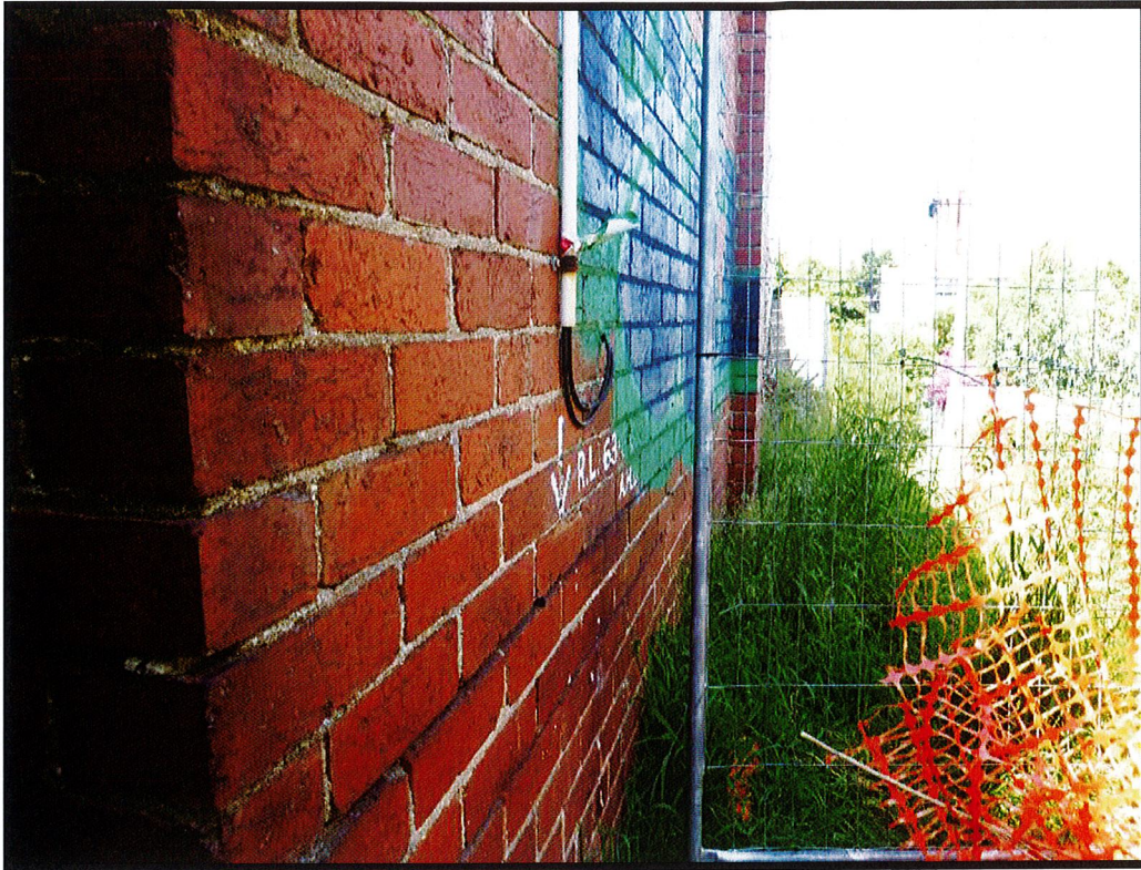
Photograph 19 – Photograph captured 19 November 2020. No evidence of movement and / or damage to the brickwork wall along the south boundary of 42 James Street, at the top of the battered ground to the subject land.
