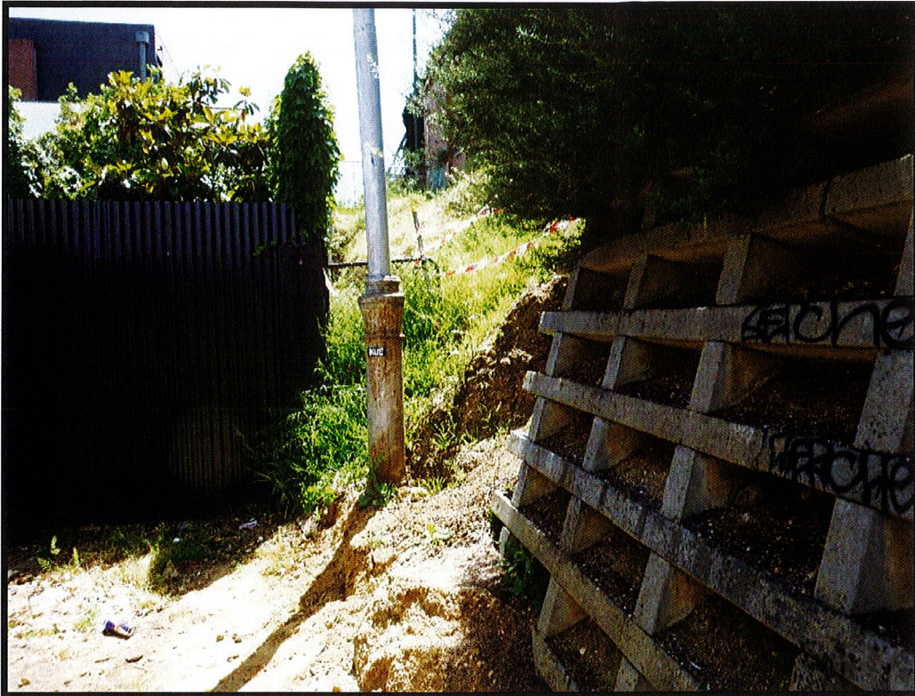
Photograph 3 – Photograph captured 19 November 2020. View of eastern end of subject land, looking west. Note spoil / loose material in laneway at the bottom of the batter. Slight erosion of material when compared to April 2019 (photograph 2).
