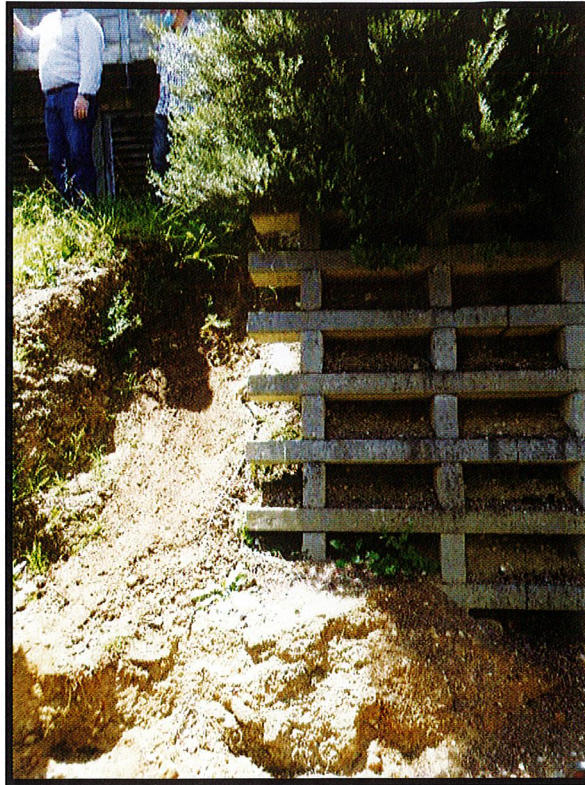
Photograph 5 – Photograph captured 19 November 2020. View of the eastern end of the subject land, looking north. Note localised erosion of land resulting in steep slope adjacent to crib wall.
