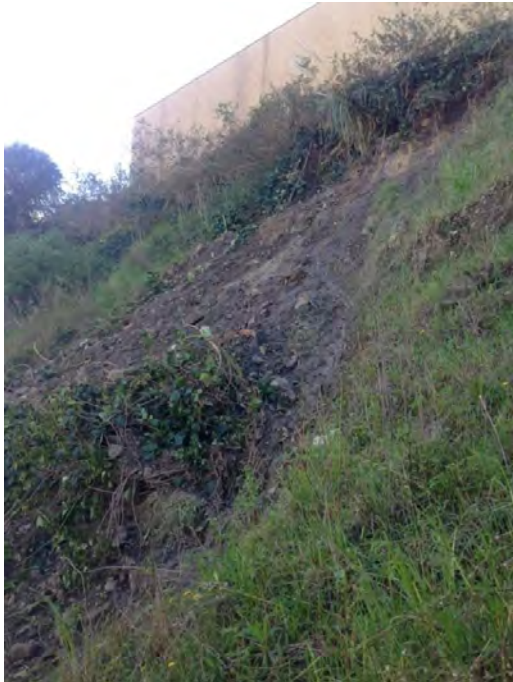
Figure 2 Fill embankment looking west showing the landslide (6 th May 2015)
