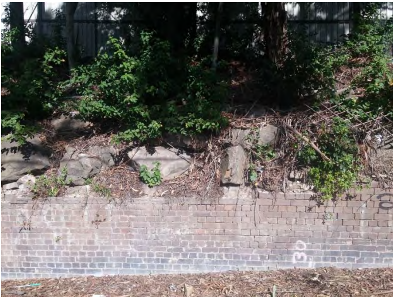
Plate 4-4 - View looking boulders just above the gravity wall on Campbell Lane
