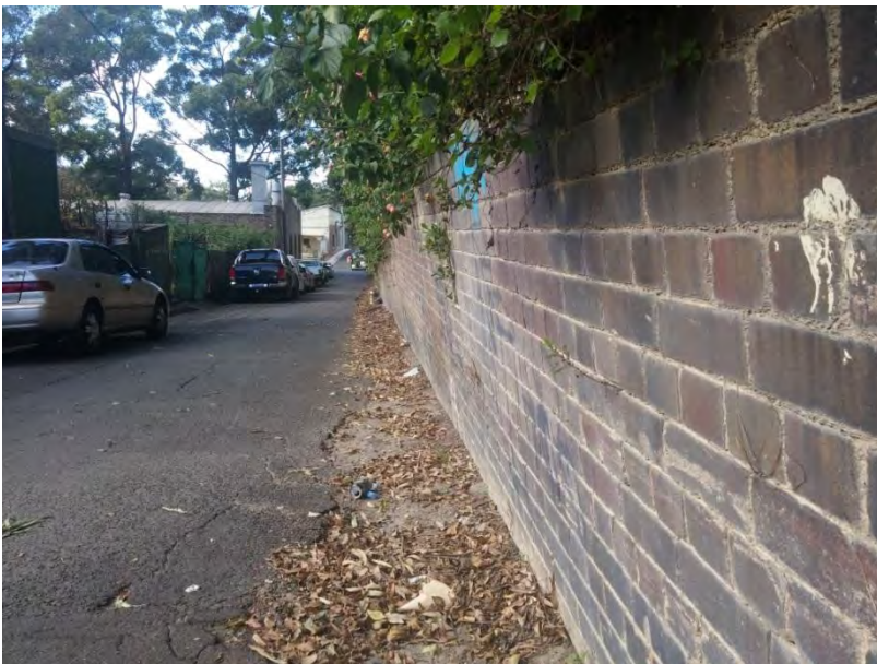
Plate 4-2 - View looking east at leaning gravity wall down Campbell Lane
