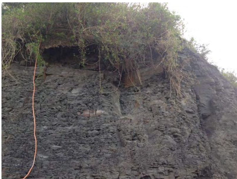
Plate 3-8 – Talus build-up (spalling, small blocks and bricks)
