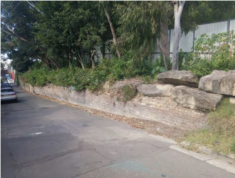
Plate 4-2 - View looking east at leaning gravity wall down Campbell Lane
