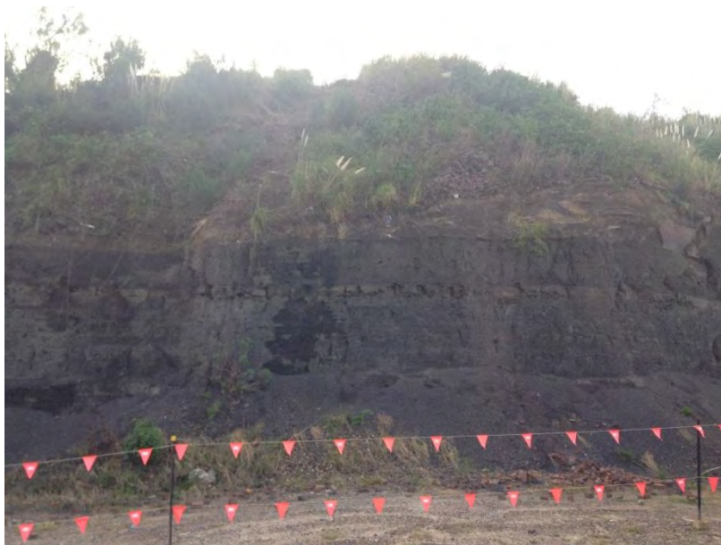
Plate 3-3 - View looking north at exposed quarry face with fill overlying the weathered shale and seepage from bedding
