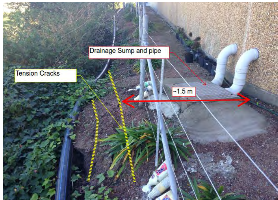
Figure 5 Crest of slope, showing tension cracks and drainage sump and pipe (20 th May 2015)
