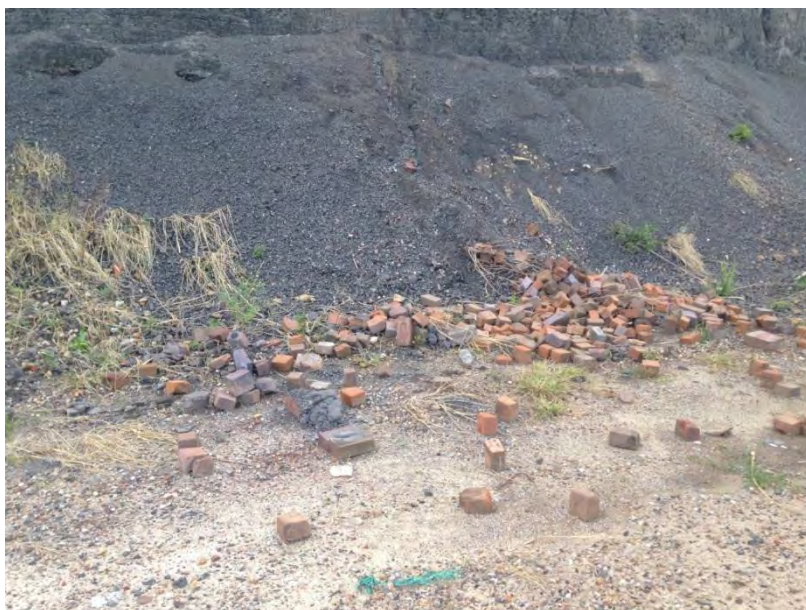
Plate 3-4 – Talus build-up and fill (bricks) at the base of the slope
