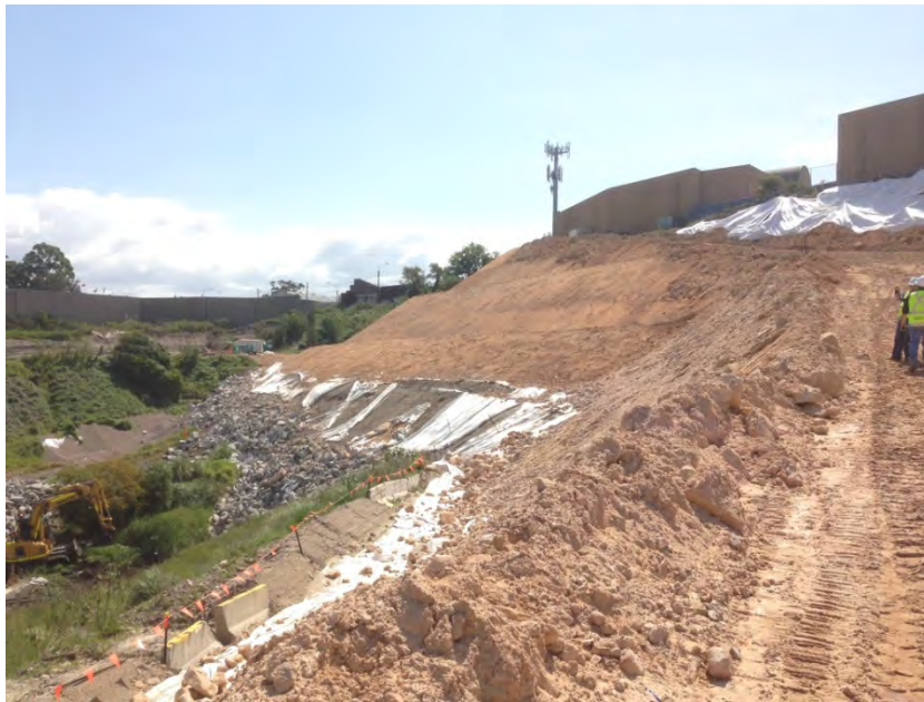
Figure 11 Construction of Temporary Stabilisation Buttress – 14 October 2015.
