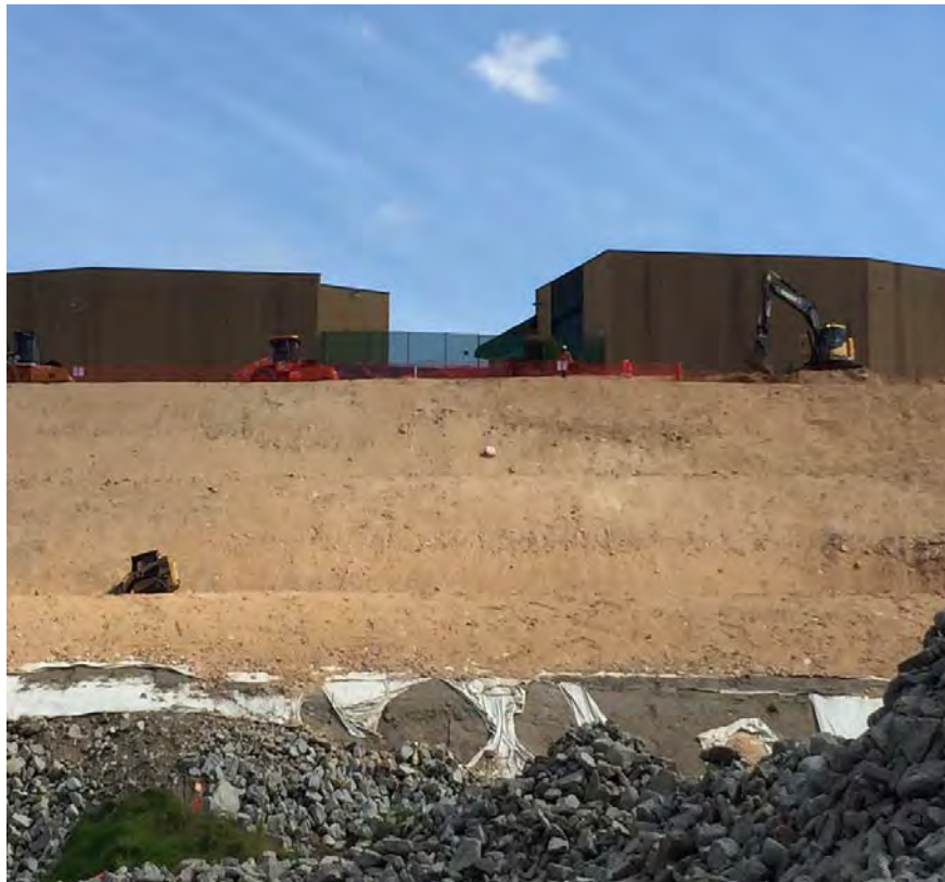
Landslip stabilisation works – earthworks complete
