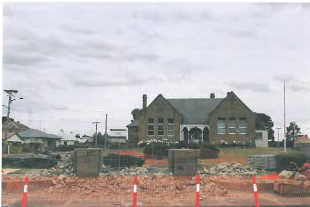
The arch in the process of removal December 2012
