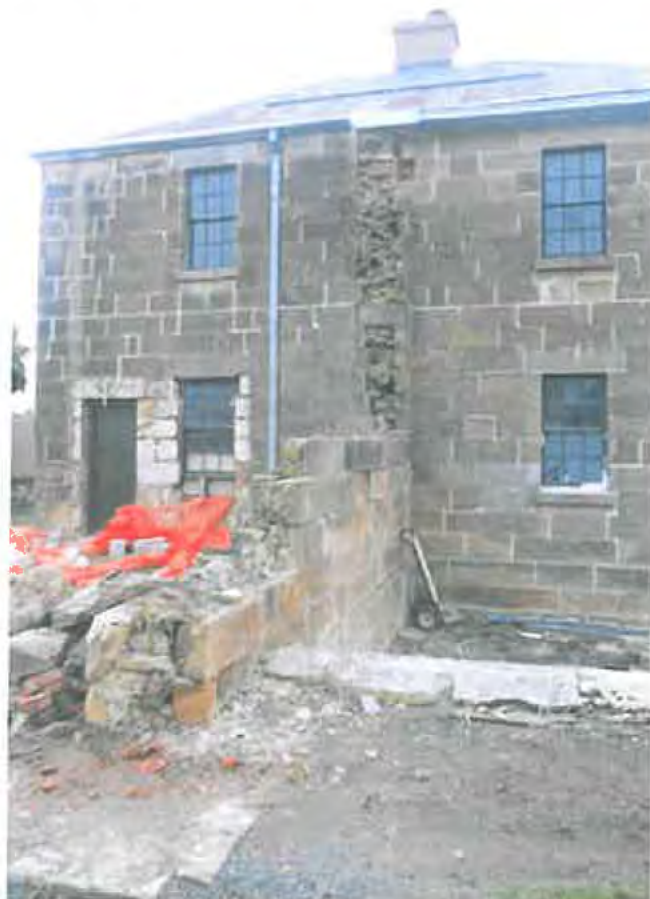
Damage to the Gaoler's Residence and remainder of walls following relocation of the arch
