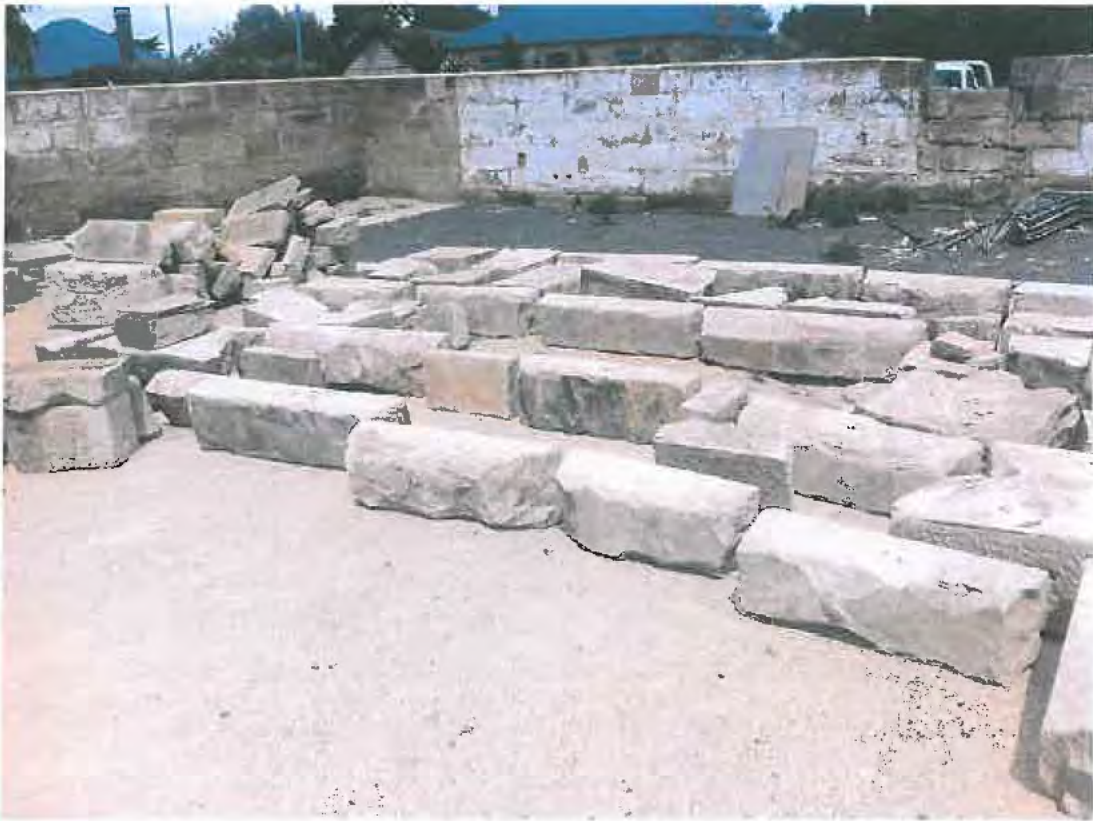
The arch laid out ready for reconstruction February 2013
