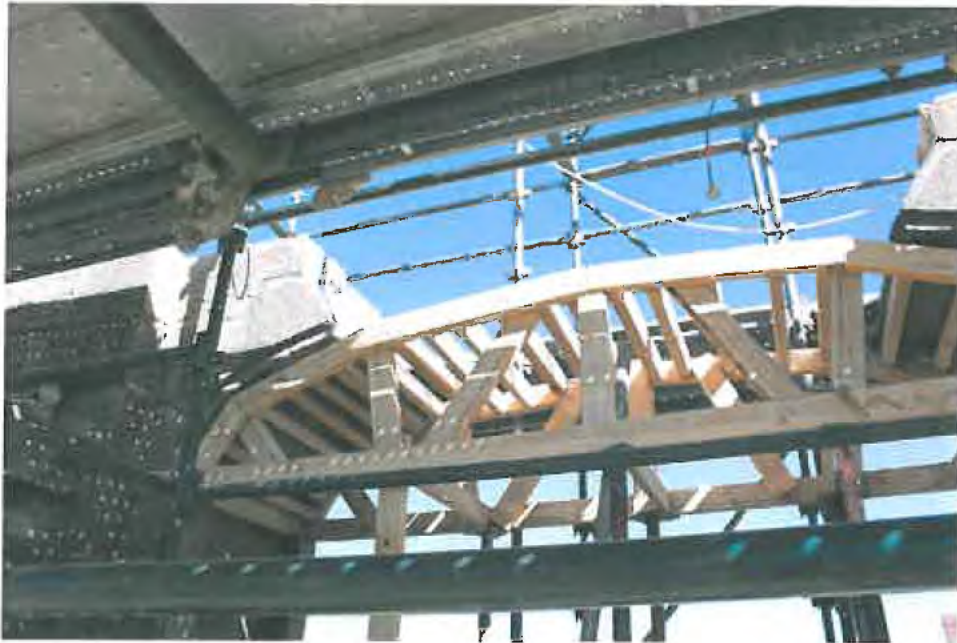
Careful reinstatement of keystones September 2013
