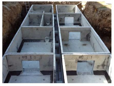
Figure 6-3 Below ground concrete detention tanks (image from www.australiantanks.com.au)
